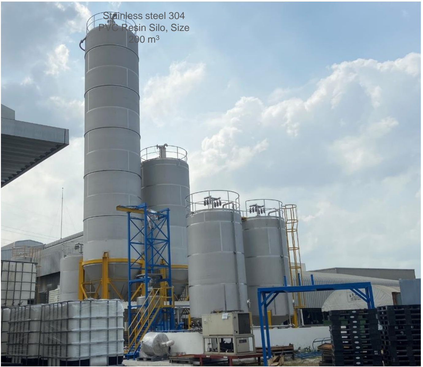
PVC Powder Silo loading & Weighting system / deliver from 16 tons bulk truck
