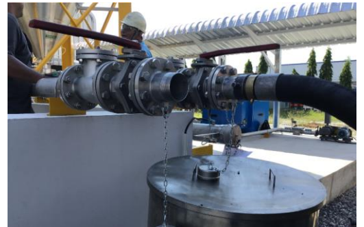
Stainless steel 304 DOA & DOTP Tanks Size 30 m 3 With the Loading in and Pumping Out System arrangement
