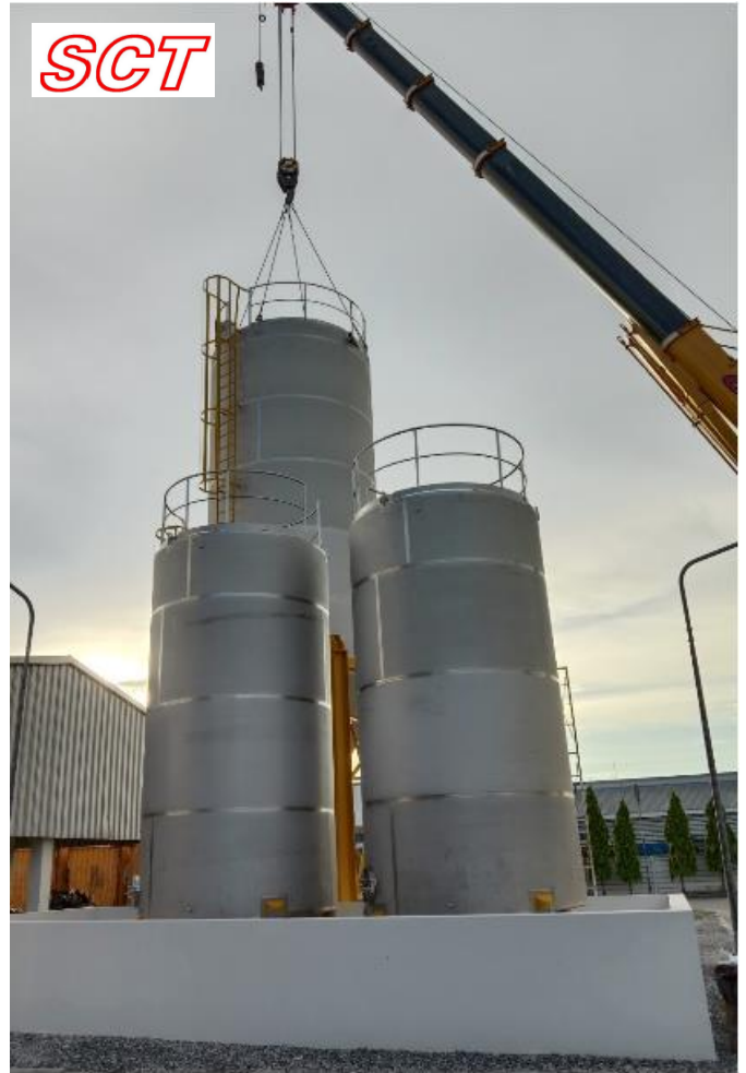
Stainless steel 304 DOA Storage Tank, Size 34 m 3
