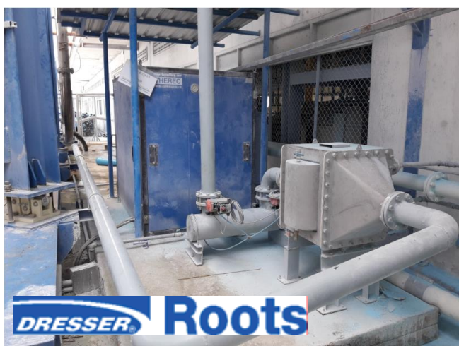
High pressure Roots blower Package with Acoustic Enclosure for PVC Bulk truck to Silo loading line with air cooler unit
