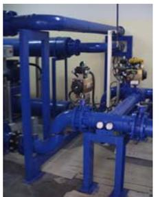
Enclosures ,Silencer, In line filter ,Control valve, All installed in the blower room
